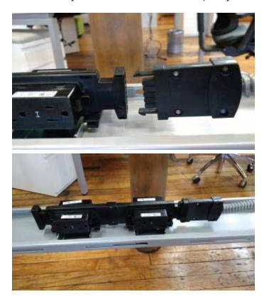
When power bars are in the desired location install the 4 securing screws that came with the cable tray.
