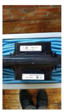
Center legs are cut out in the middle to allow cables to pass through to the next tray
