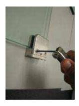
Secure the Flat Head Screws for Maximum Clamping Strength
