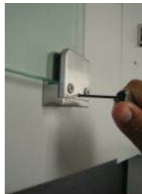
Slightly tighten the Allen Screw so the Plate tilts at a slant
